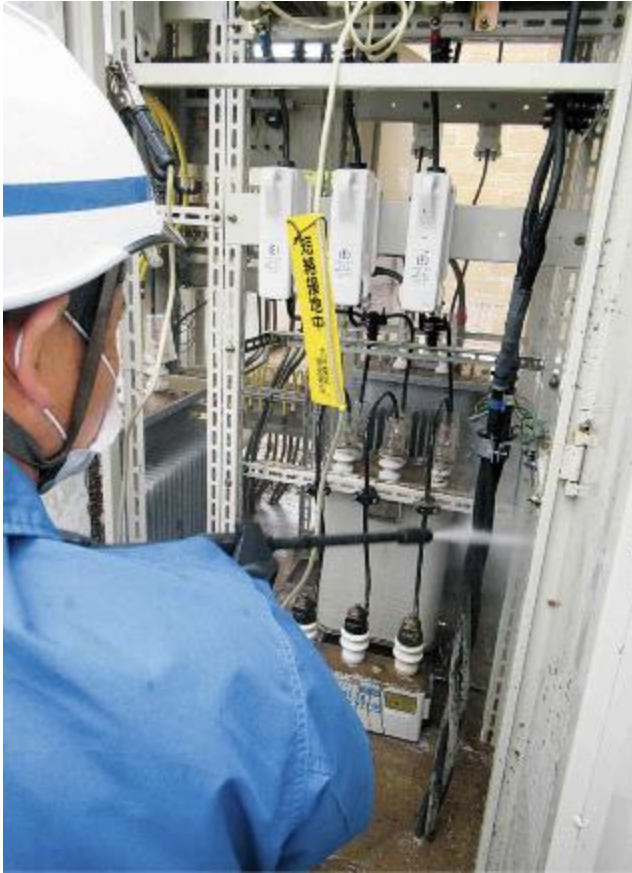
[Cleaning of a flooded electrical facility]
