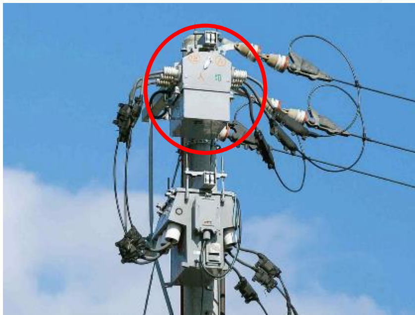
[Installation of a switching device with a built-in lightning arrester]
