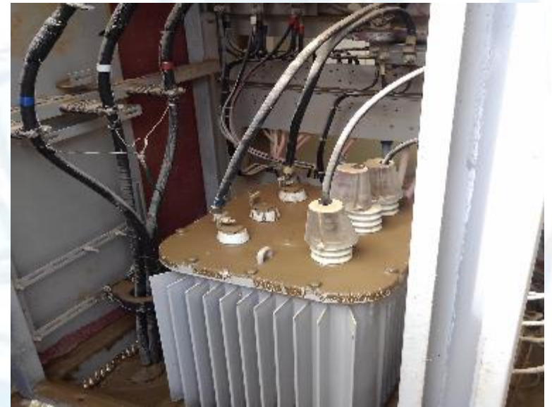
[Flooded transformer]
