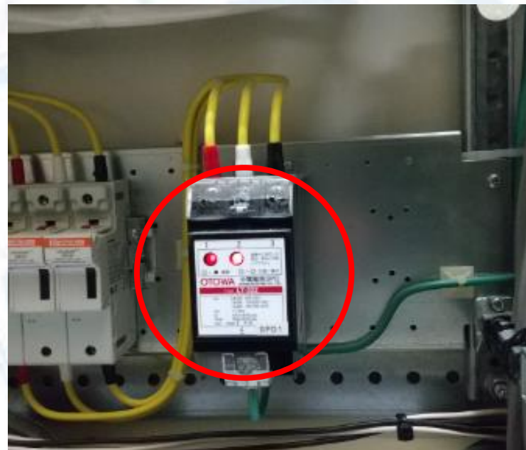
[Installation of a lightning arrester in the low-voltage circuit]
