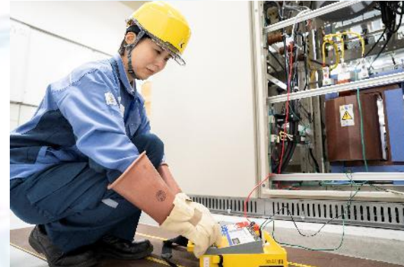
Inspection with power outage
