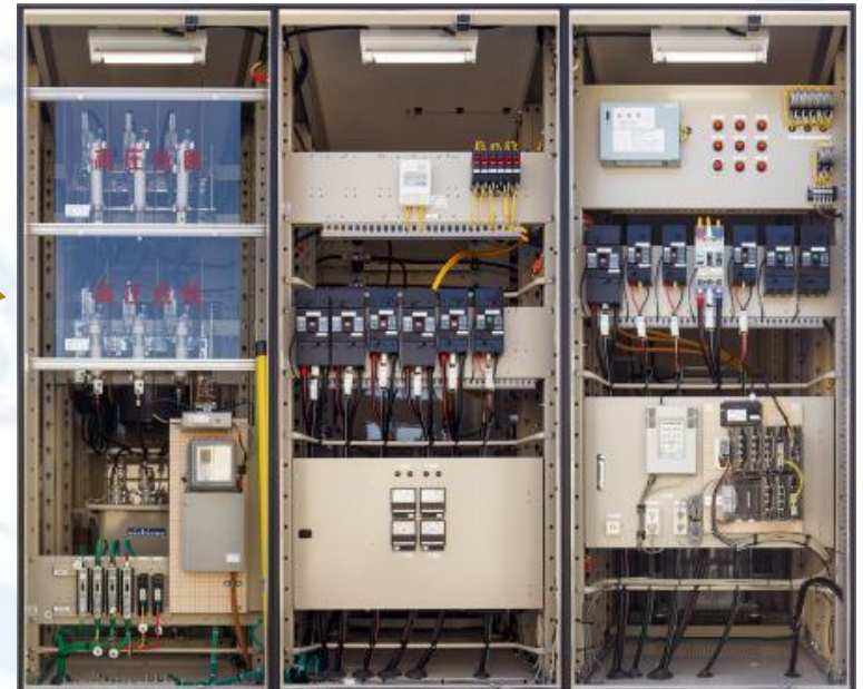
Inside of the cubicle
