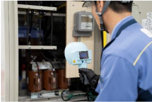
Inspection without power outage
