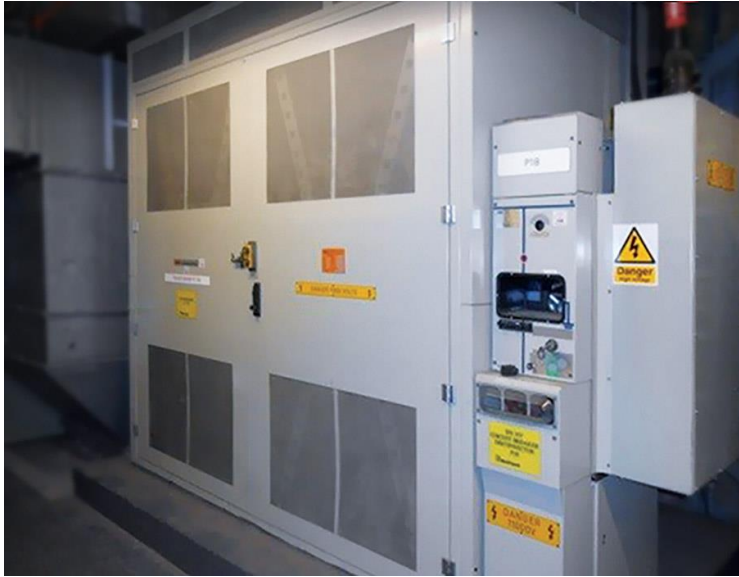
An example of a 2000 KVA 11KV-415v cast resin transformer
