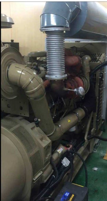
Emergency Diesel Generator
