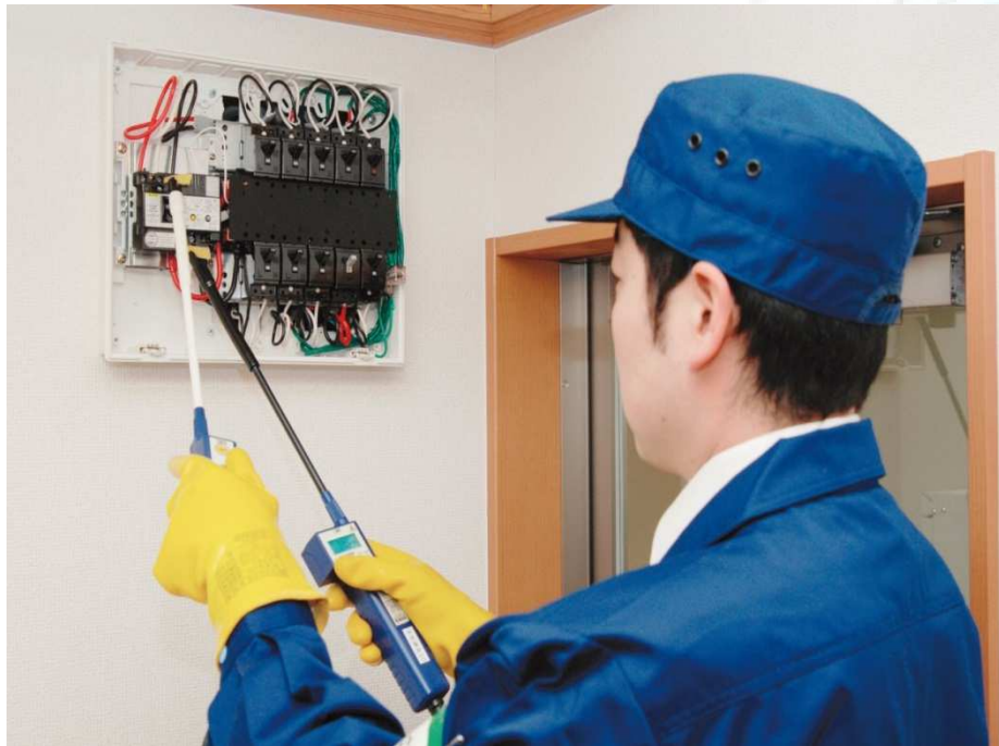
Insulation resistance measurement
