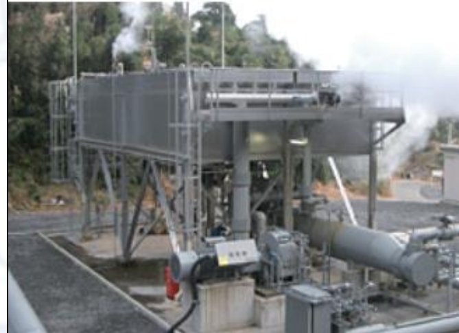
Example of facility in a hot spring resort that uses geothermal steam to drive turbines
